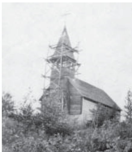
Photo: Longville Church -- under construction in 1920.
